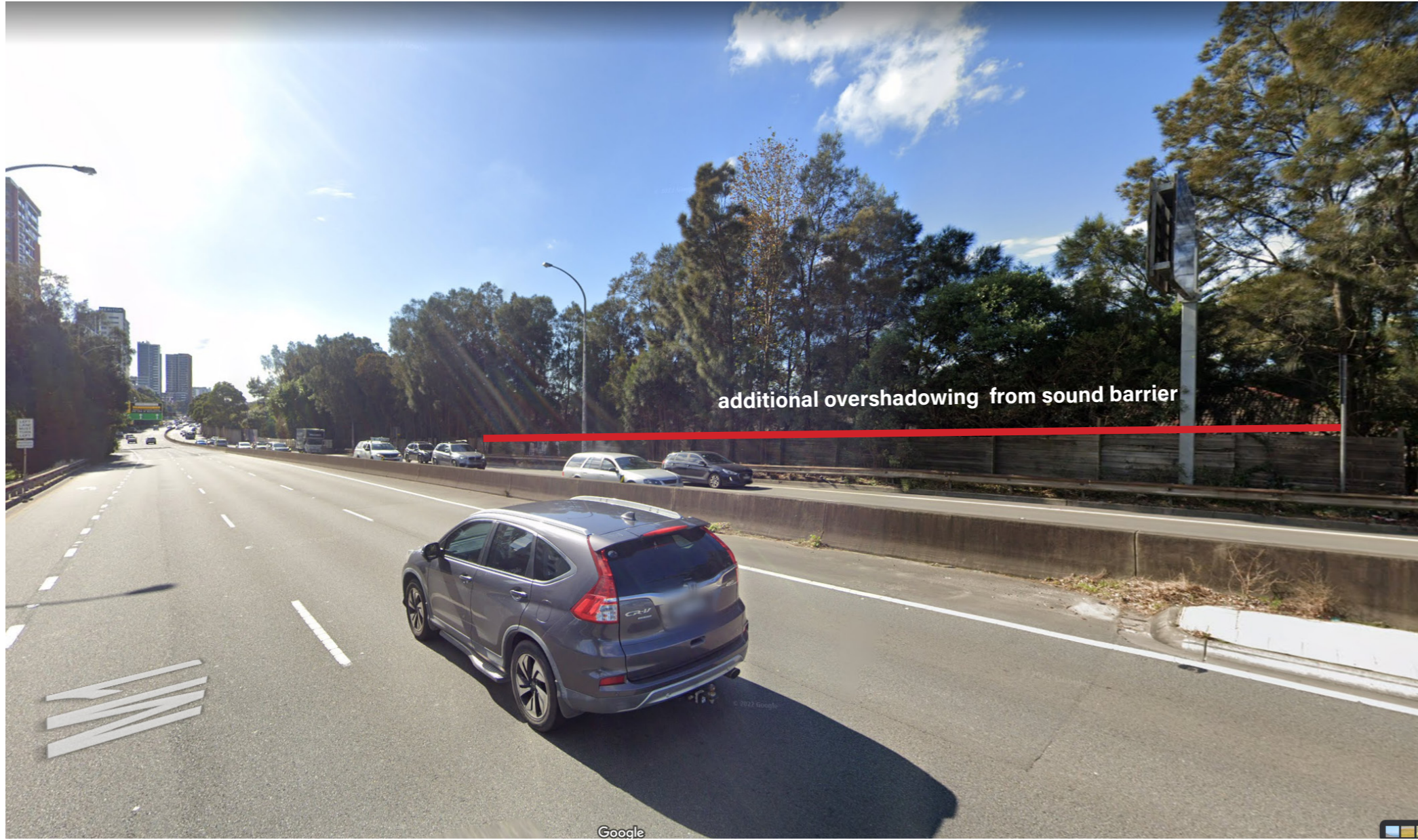
a) View of Sound Barrier on Southern Cross Drive
